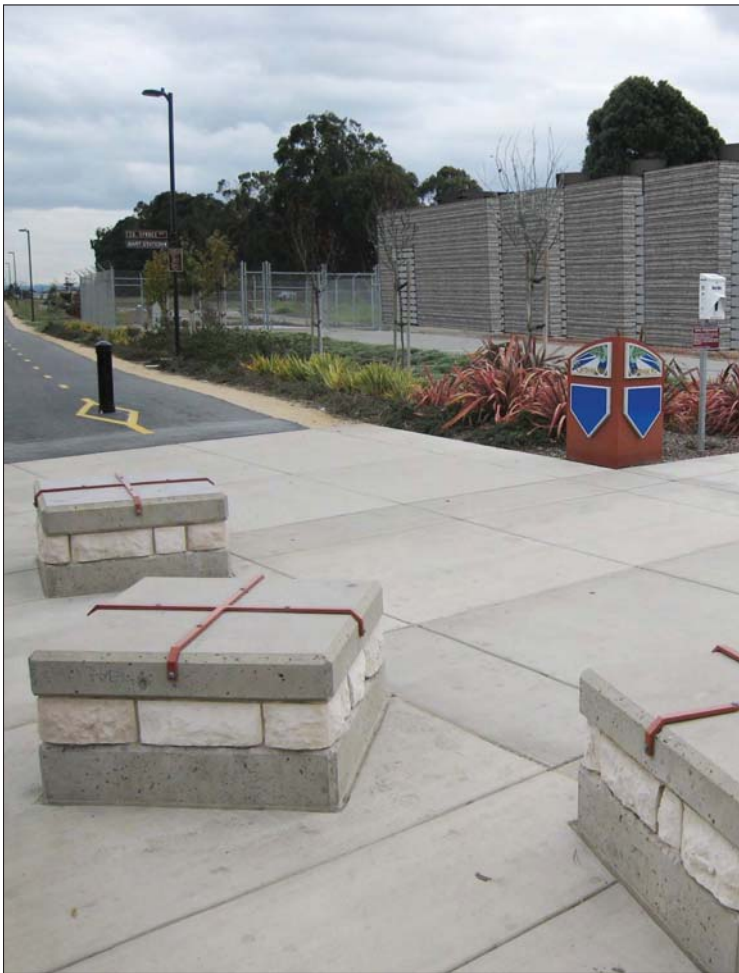
▲ Golden Gate Park Groundwater Supply Well Stations
