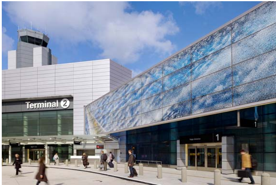
North façade (detail).
