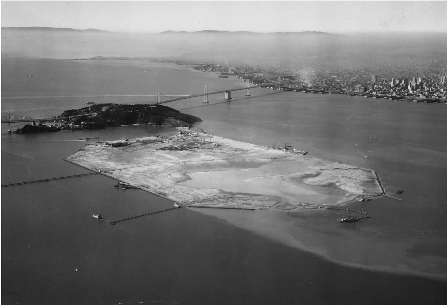
Figure 1.03 The Construction of Treasure Island
